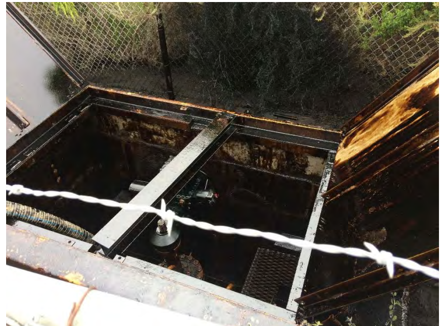
Valve Flange leak in Vault (500-1000 barrels during start up)
