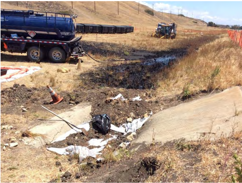
Static Drain Down – (3000 barrels while line idled)
