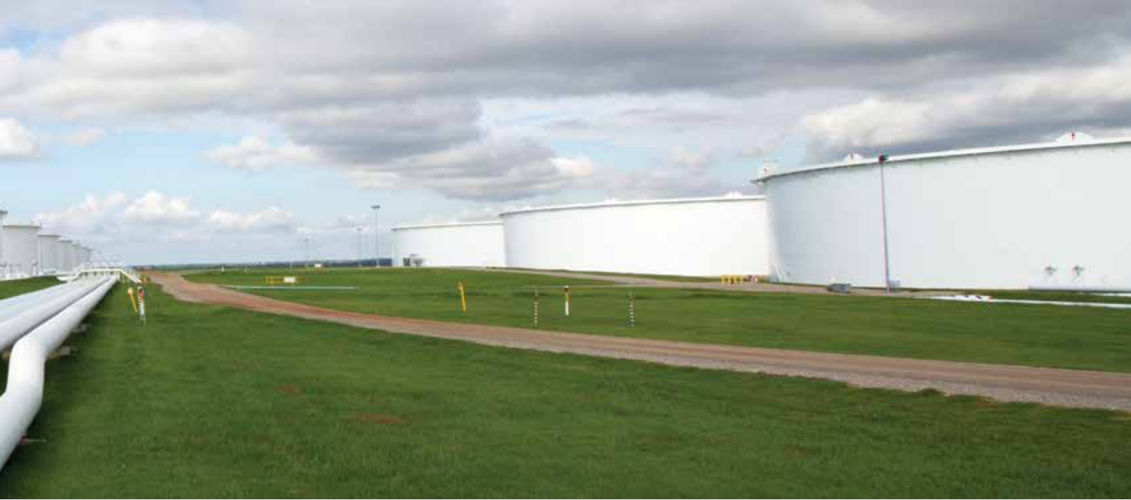
Photo courtesy of Plains All American Pipeline
